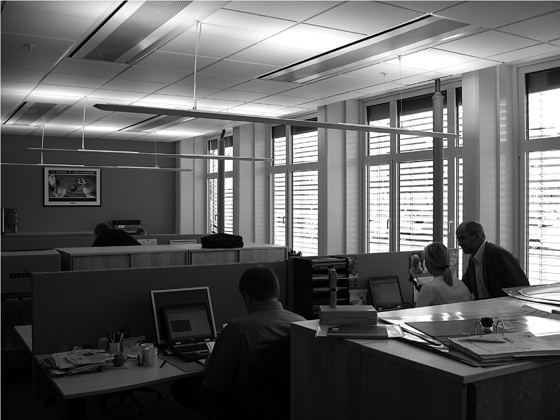
Figure 3. In the office landscape the luminaires were positioned parallel to the length of the tables providing only indirect lighting. Notes. Luminance from the ceiling was 600–800 \text{cd}/\text{m}^2 .
