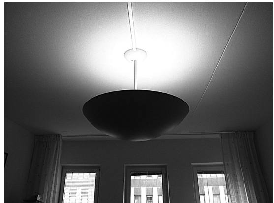
Figure 2. In a few single-occupancy offices the luminaire was disc-shaped, suspended 30 cm from the ceiling. Notes. Four lighting tubes were lit upwards giving luminance from the ceiling of 1500\text{--}1800 \text{ cd/m}^2 .
