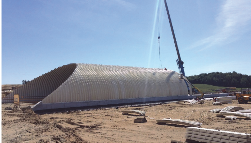
Figure 3. Structure during assembly
