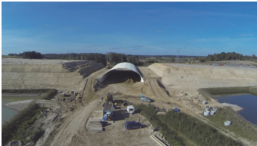
Figure 4. Structure during backfilling
