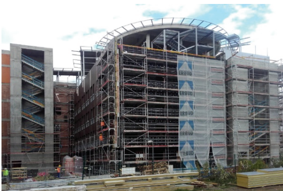
Fig. 2. Helipad on top of a building frame (e.g., Warsaw South Hospital) and a design scheme
