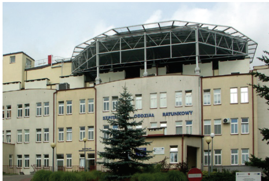
Fig. 3. Helipad on a rooftop of an existing building (e.g., hospital in Iława) and a design scheme
