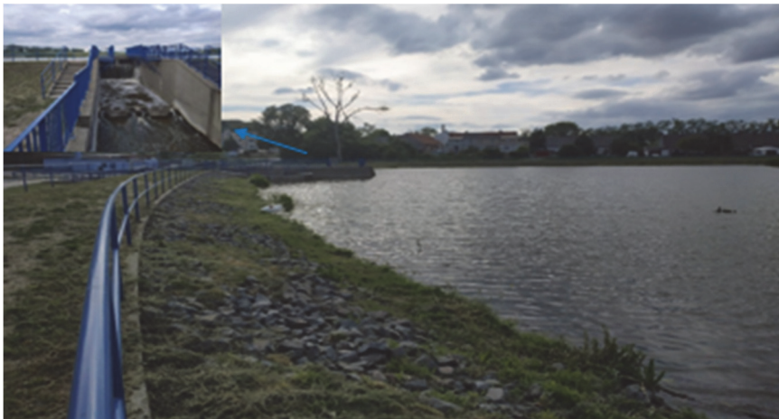
Fig. 2. The embankment dam with the spillway-overflow structure (steady level damming) in the Przebédowo reservoir
