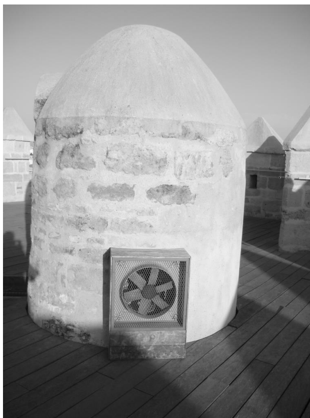
Fig. 2. The ventilator on the tower of old Moorish castle (photo K. Gładyszewska-Fiedoruk).
