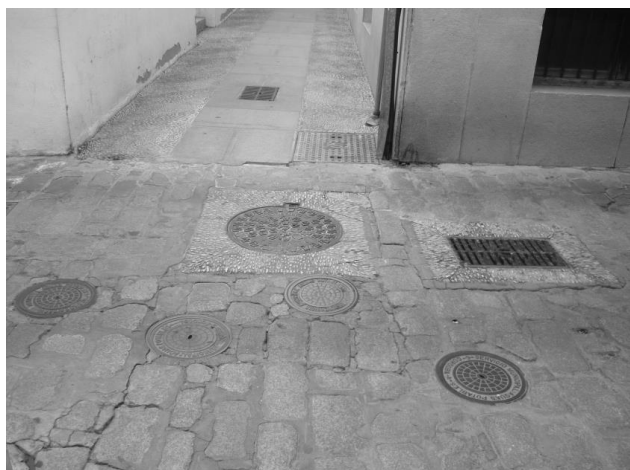
Fig. 7. The manners of street sink basins and inspection chambers (photo A. Rodero Serrano).
