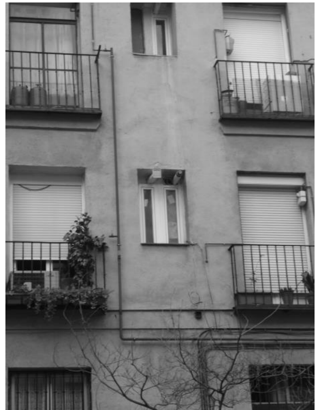
Fig. 6. The conductors and other pipes in Madrid (photo D.A. Krawczyk).
