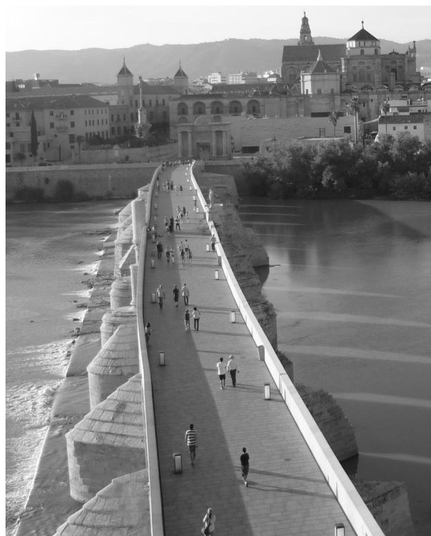
Fig. 10. The street lamps on the ancient bridge in Cordoba (photo K. Gładyszewska-Fiedoruk).
