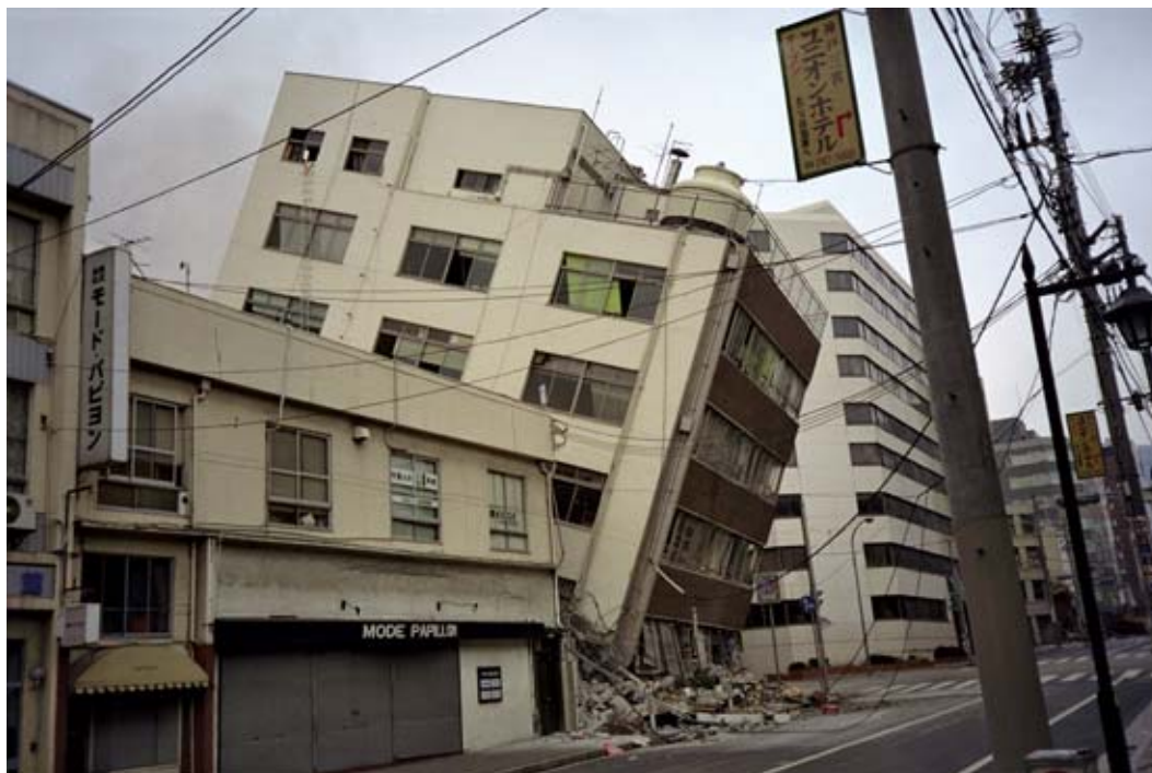
Fig. 4. Earthquake damage. Source: Fot. Dr. Roger Hutchison/NGDC [17]
