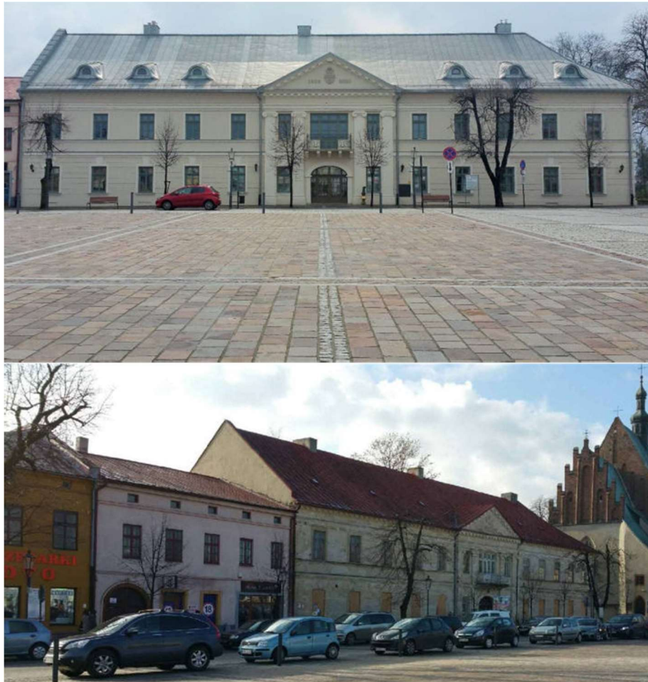
Fig. 2. Main façade, view from the Market Square, after and before renovation (Photo by the author)
