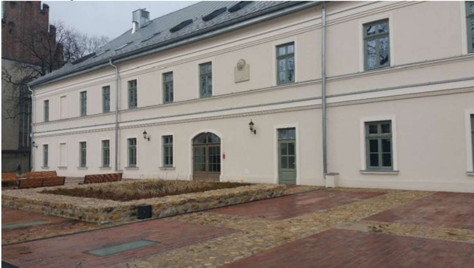
Fig. 5. Façade seen from the courtyard. After renovation (Photo by the author)
