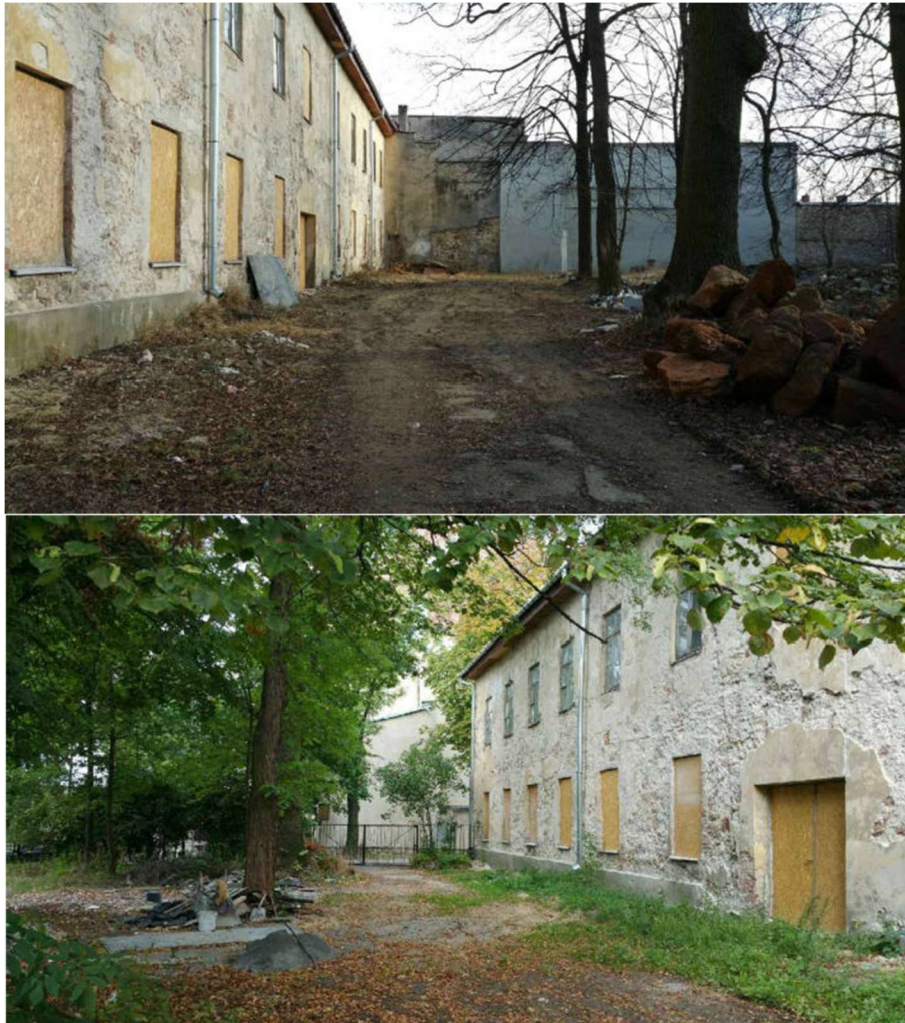
Fig. 4. Façade seen from the courtyard. Before renovation (Photo by the author)
