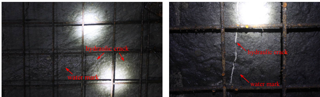
(a) Fracture morphology
