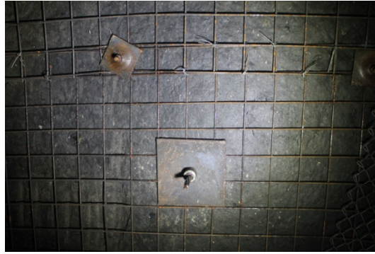
Fig. 2. Integrity of coal seam roof
