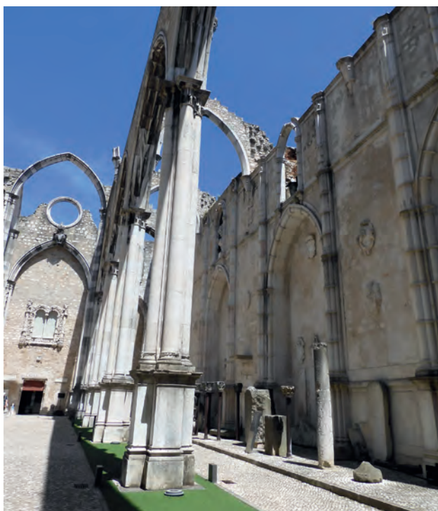
Figure 5. The corps of the church – Igreja do Carmo, 2021, photo: M. Doroz-Turek
