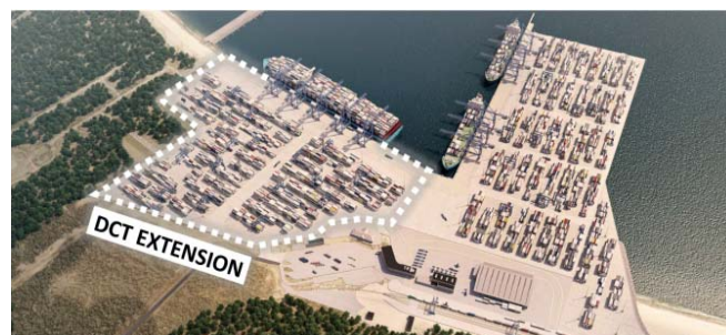
Fig. 3. Bird view of the new quay wall and container storage yards (acc. DCT Gdańsk S.A.)
