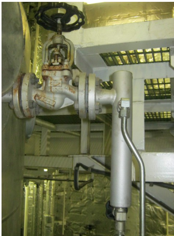
Fig. 2. Water level sensors assembled on the selected smoke-tube exhaust gas boiler
