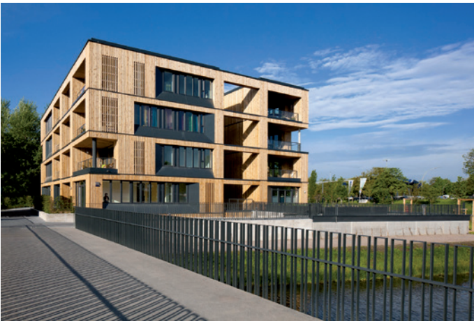
ii. 4. The 'Hybrid Development' wooden structure condo (photo courtesy of Bieling Architekten)
