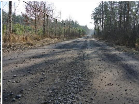
e) view of the test track section classified as a destroyed concrete road
