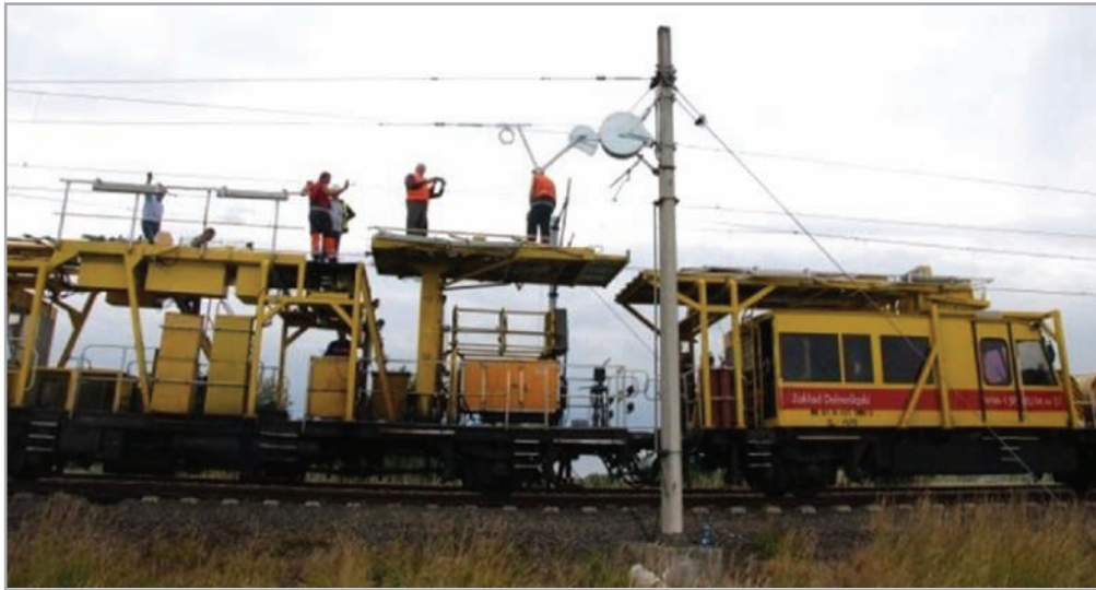
Fig. 31. Assembly of the no-load tensioning device [photo P. Kwaśniewski]
