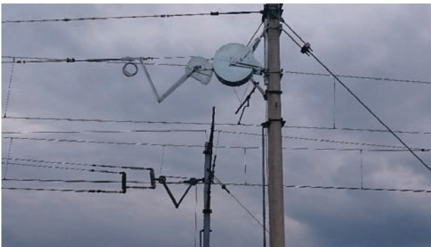
Fig. 32. Mounted no-load tensioning devices. Commonly used tensioning device with loads is visible in the background [photo A. Rojek]
