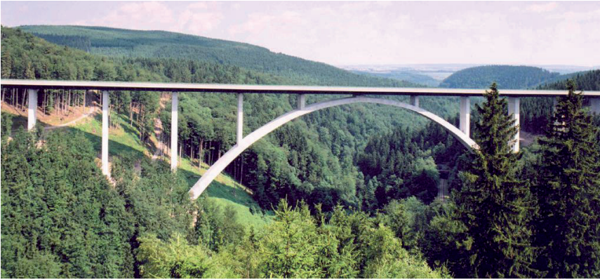
Fig. 2. The Wilde Gera bridge ( http://www.highestbridges.com/wiki/images/f/1WildeGeraBridge.jpg ).
