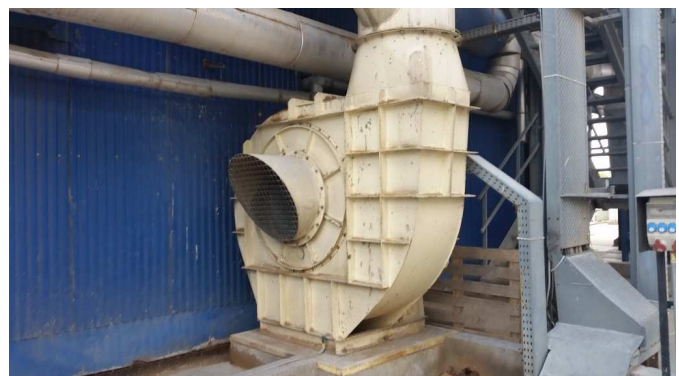
Fig. 4. Source Z1 (industrial fan) – flow Q = 28\,500\text{ m}^3/\text{h} , diameter 0.7 m, frequency range 800–920 Hz.
