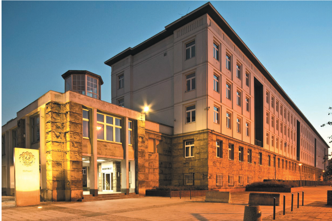
Fig. 4. View of the Faculty of Mining, Safety Engineering, and Industrial Automation (from the Rector's Office)
