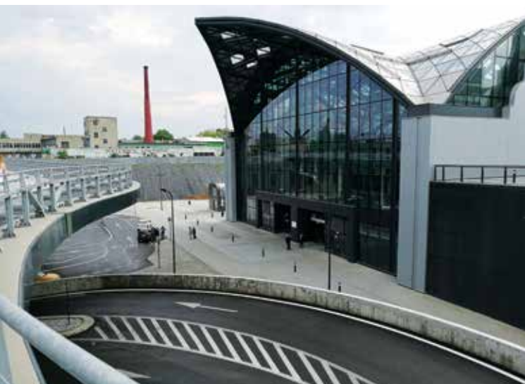
Entrance to the station from the east
