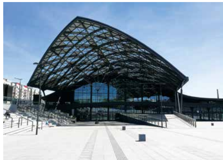
Entrance to the station from the west
