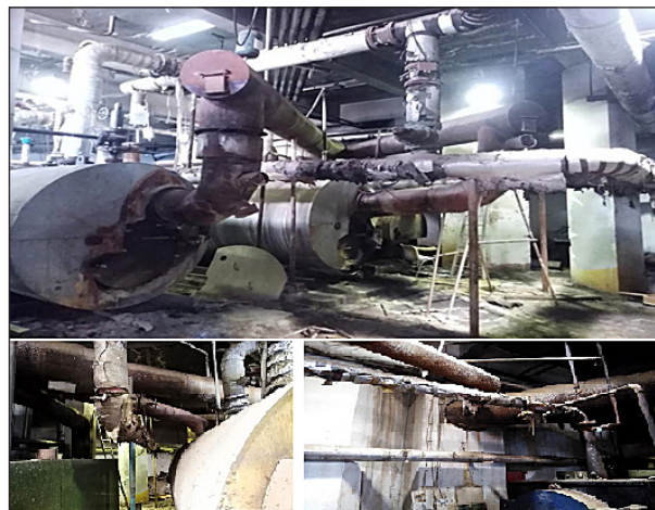
Figure 6. Pipe insulations evaluation
