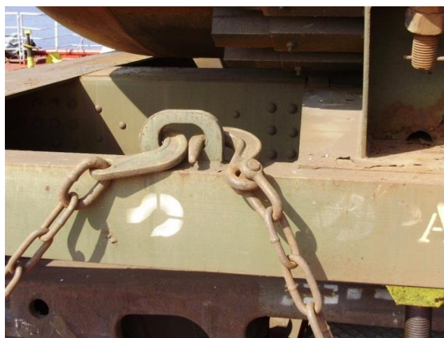
Figure 7. The scheme of fixing the tank wagon relative to the railway ferry deck
