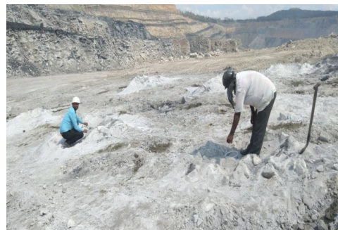
Fig. 4. Burden &amp; spacing measurement
