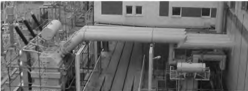
Fig. 1. Isolated phase busduct [5]
