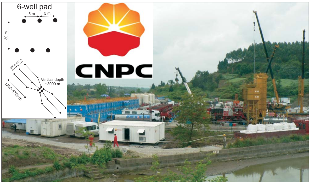
Fig. 4. Multi-well pad W202H2, Weiyuan block, Sichuan, operated by the CNPC Company. The picture shows the 6-well pad. Photo by G. Pieńkowski
