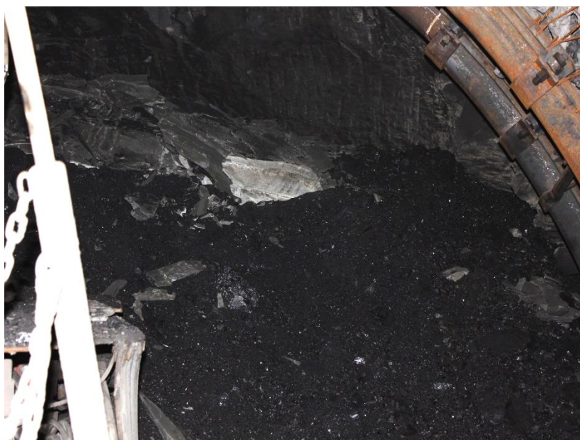
Fig. 5 Heading face after the outburst of gases and rocks in ramp D in seam 358/1 (11.05.2012)
