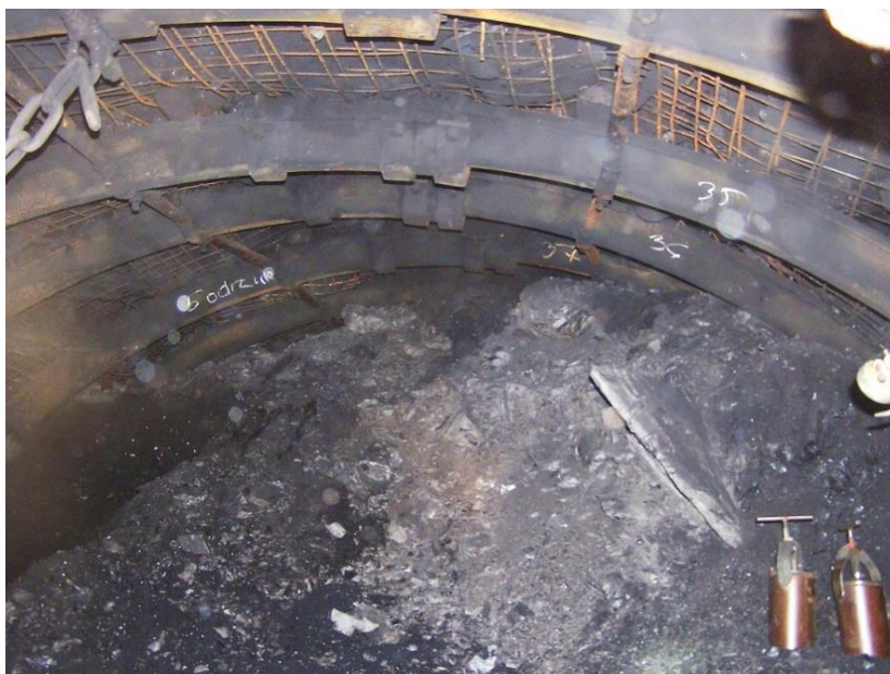
Fig. 1 Heading face after the outburst of gases and rocks in transport gallery D-6, seam 409/4 – "Zofiówka" mine (November 22, 2005)
