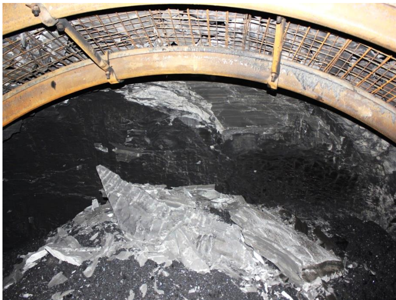
Fig. 4 Heading face after the outburst of gases and rocks in ramp D in seam 358/1 (11.05.2012)
