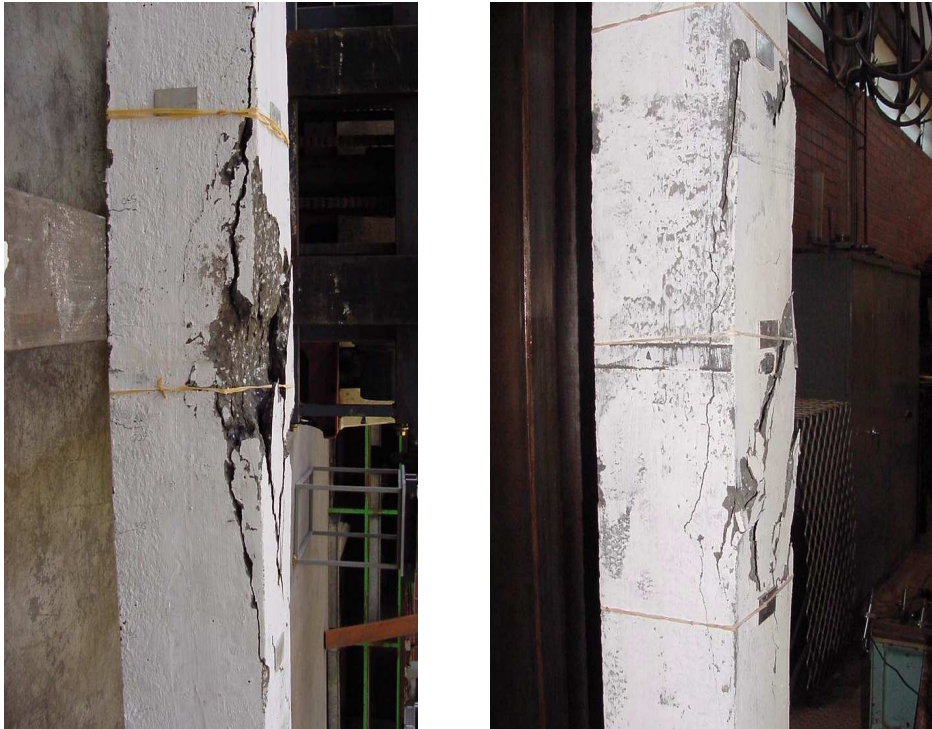
Fig. 11. Example of reinforced concrete pillars from geopolymeric concrete after the performed durability tests [28]
