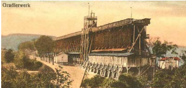
Fig. 3. – Section of a postcard from 1928 showing the graduation tower of Kösen on the Rechenberg. The framework has a length of 320 m.
