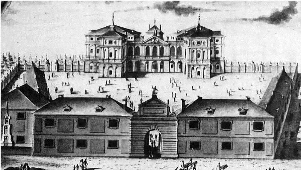
Fig. 4. Andrzej Morsztyn's manor house before the 1712 decision by King August II to expand it. (view from Krakowskie Przedmieście Street (lit. 'The Kraków Suburb') as in a figure from the era). Source: available in the public domain
