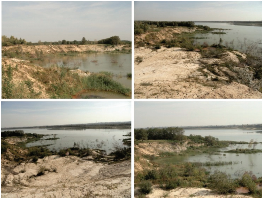
Fig. 1. State of the slope after the formation of the landslide (Source: photo by J. Jakóbczyk)
