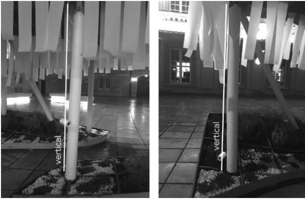
Figure 11. Position of the columns
