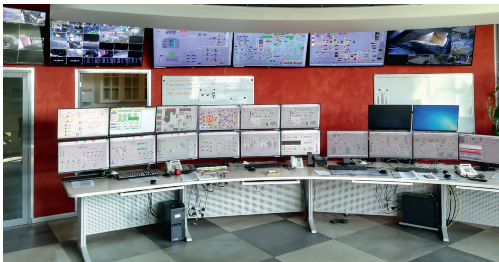
Photo 3. Fragment of a modern DCS MASTER control room with LCD monitors and a touch panel
