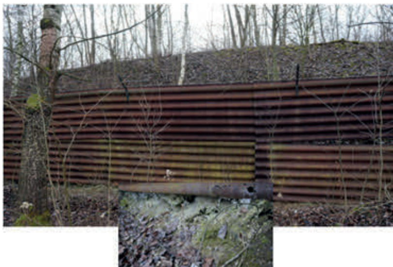
Fig.6. Fragment of fencing at facility heap. Szczucin 2013 [M. Glica]
