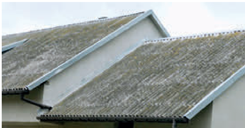
Fig.4. Eternit roofing (Szczucin, 2013) [M. Glica]
