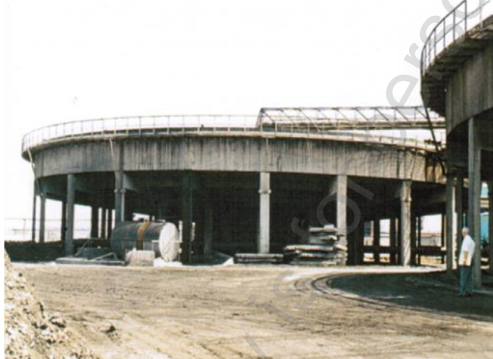
Fig. 4. Structural damage to the elevated Dorr's clarifier at Huta Miedzi (copper smelting plant) [4]: a) vertical cross-section of the clarifier, b) plan of the clarifier, c) general view of the clarifier, d) view of the clarifier filled with sludge
