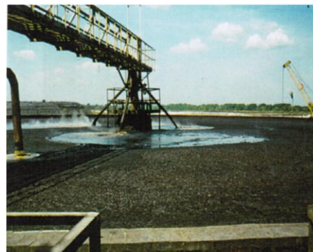
Fig. 4. Structural damage to the elevated Dorr's clarifier at Huta Miedzi (copper smelting plant) [4]: a) vertical cross-section of the clarifier, b) plan of the clarifier, c) general view of the clarifier, d) view of the clarifier filled with sludge
