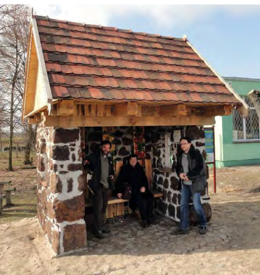
Fig. 11. The bus stop shelter, made from a bog ore in Górne Grądy (photo by H. Zaniewska, 2013)
