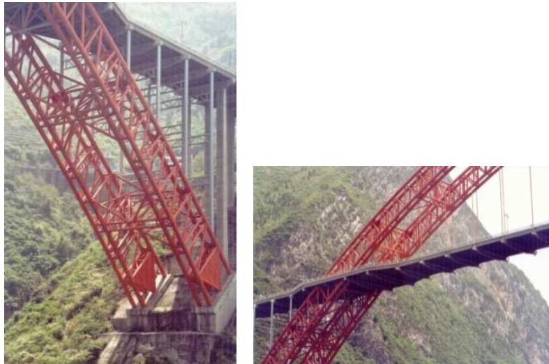
Fig. 25. Tubular concrete structure (CFST) of arch road bridge over the Yangtze river, Wushan, China, 2005 (460 m)
