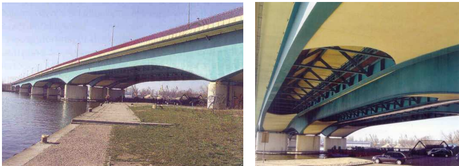
Fig. 12. Girder bridge of double composition over the Regalica river in Szczecin (Poland)
