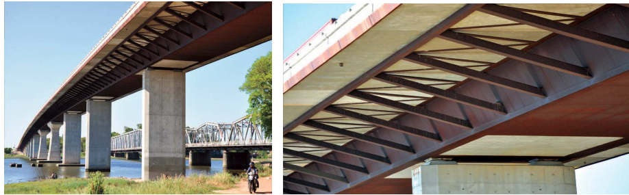
Fig. 13. Girder bridge of double composition over the Santa Lucia in Uruguay
