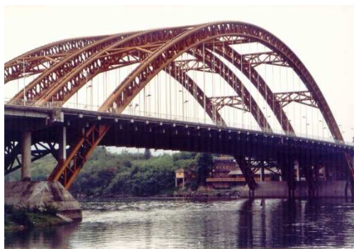
Fig. 29. Truss concrete filled steel tubular (CFST) through bridge of 200 m span, near Quilin (China)
