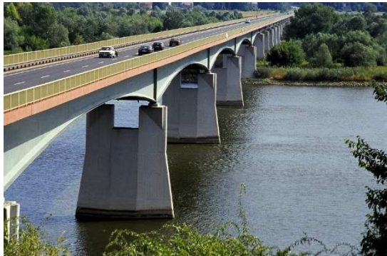
Fig. 7. Bridge over the Vistula river in Wyszogród (Poland)
