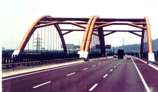
Fig. 28. Arch bridge from CFST elements along the route to Ningbo (China)
