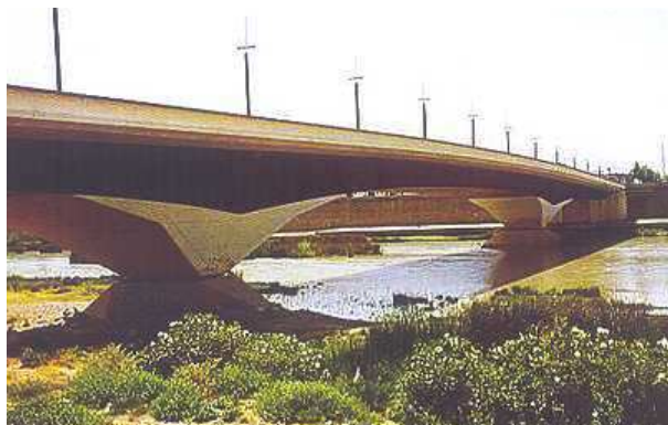
Fig. 16. Julio M. Calzon, "del Arenal" bridge over the Guadalquivir river, Cordoba, 1993 (110 m)
