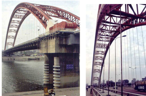
Fig. 30. Quinghuan bridge over the Han river in Wuhan (China)
