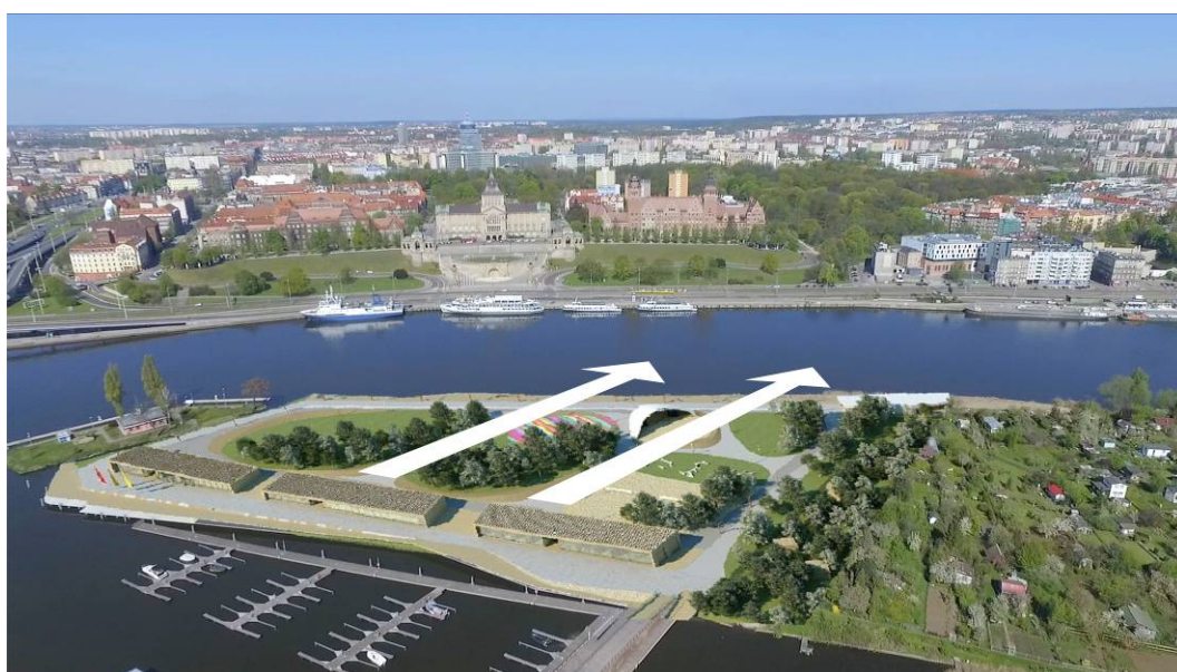
Fig. 13. Analysis of the view axes of the walkways featured by the site plan of the Szczecin Yacht Port. The analysis was performed by layering the design on top an aerial photograph of this fragment of the city. Source: original work and photograph by the author, [8]
