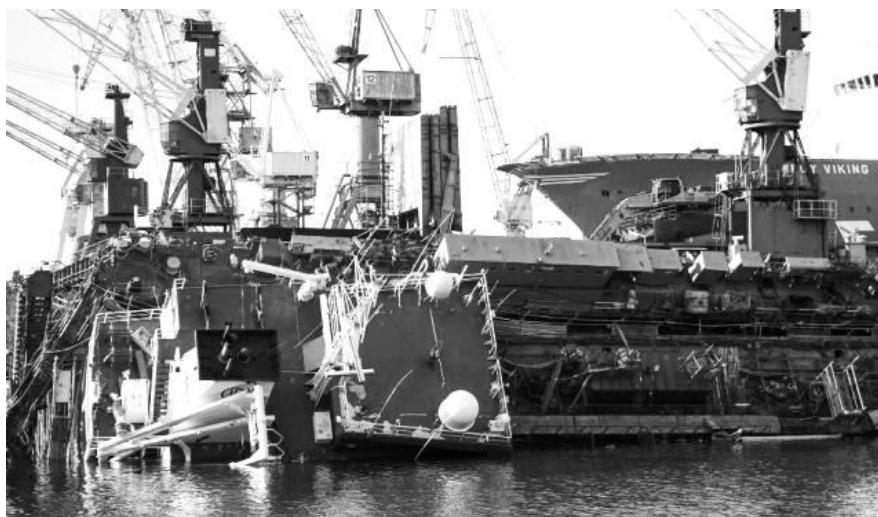
Fig. 7. Overflow dock No. 1 and the docked ship at Nauta Shiprepair Yard.
