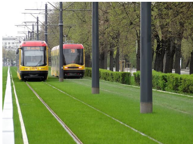
Fig. 7. Grass tram track in Warsaw [16]
