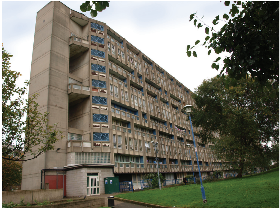
Fig. 7. Alison Smithson and Peter Smithson, Robin Hood Gardens Residential Estate in London – heavy concrete forms, 1969–1972 (photo by W. Niebrzydowski)
