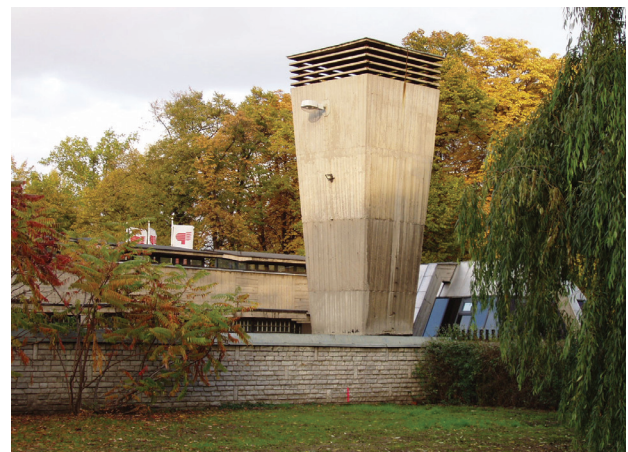
Fig. 4. Ewa Dziekońska and Marek Dziekoński, Museum of “Panorama Raclawicka” in Wrocław – exposed air exhaust chimney reflecting the principle of emphasizing technical elements, 1966–1970 (photo by W. Niebrzydowski)
