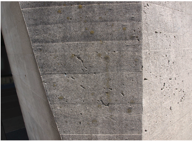
Fig. 5. Marcel Breuer, Becton Engineering and Applied Sciences Center in New Haven – defects of concrete texture as an example of preconceived imperfectionism, 1969–1970 (photo by W. Niebrzydowski)
