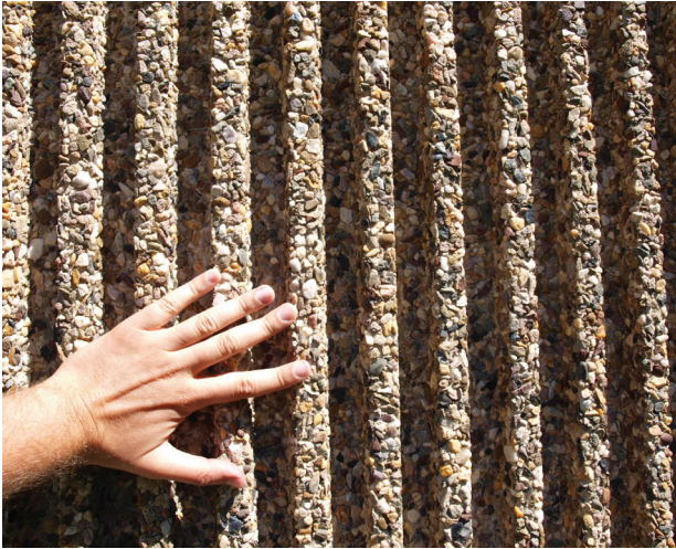
Fig. 1. Austin Arts Center in Hartford – texture of corrugated concrete as a tactile element of brutalist buildings, 1963–1964 (photo by W. Niebrzydowski)
