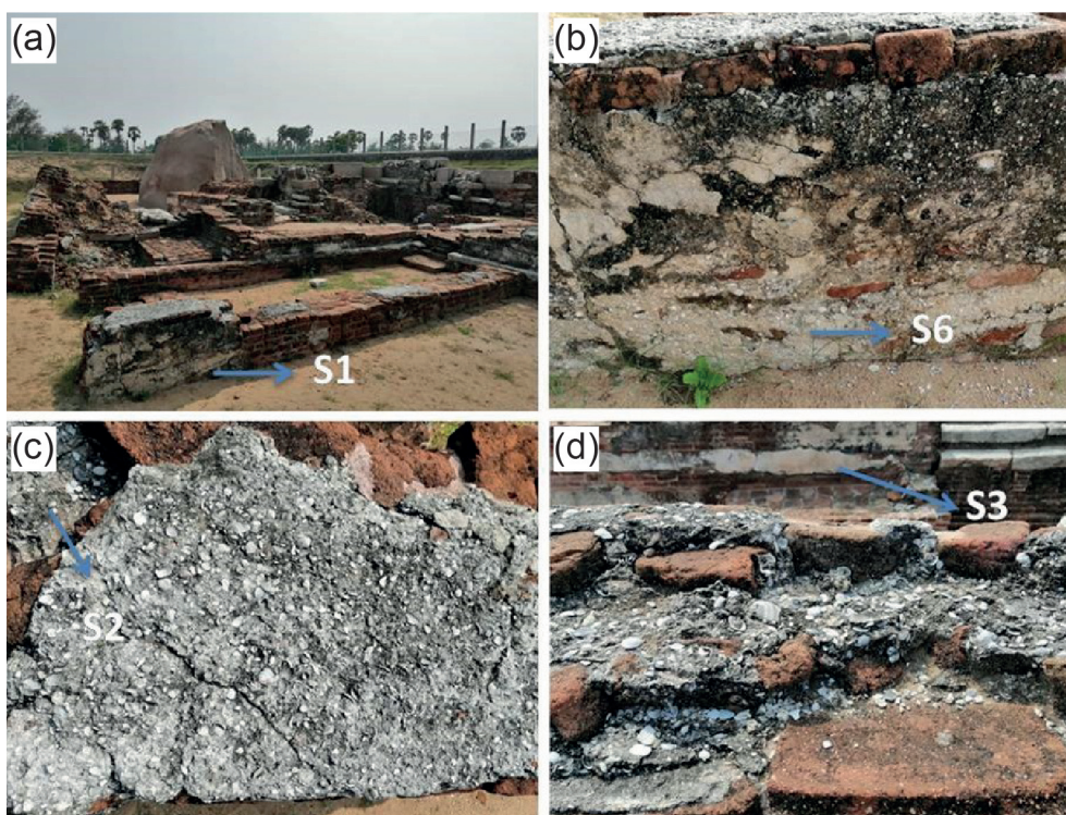
Figure 2. (a) General view of excavated temple complex of Salvankuppam; (b) lime plaster of the temple; (c) lime plaster of the temple with sea shells; (d) lime plaster of the temple with sea shells (sample collection locations mentioned with arrows).
