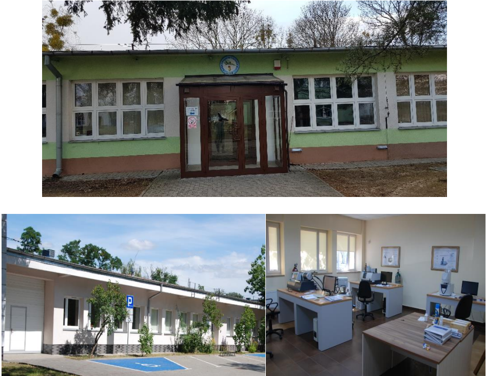
Fig. 20. View of Building 72 (DAT) and Building 66 converted into the Aerospace Propulsion Research Laboratory, with one of the rooms at the Thermal Properties Testing Laboratory
