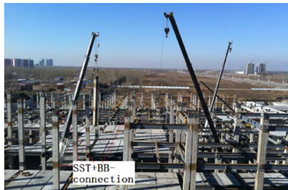
Fig. 1. SSPBB connection in practical project
