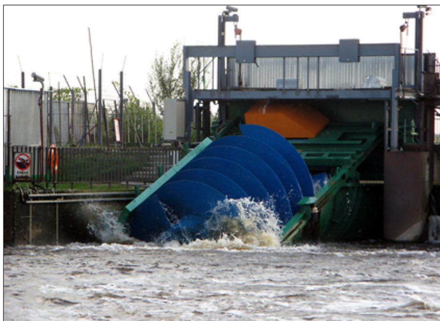
Fig. 8. First in Poland Archimedes screw turbine on the Radomka river [11]
