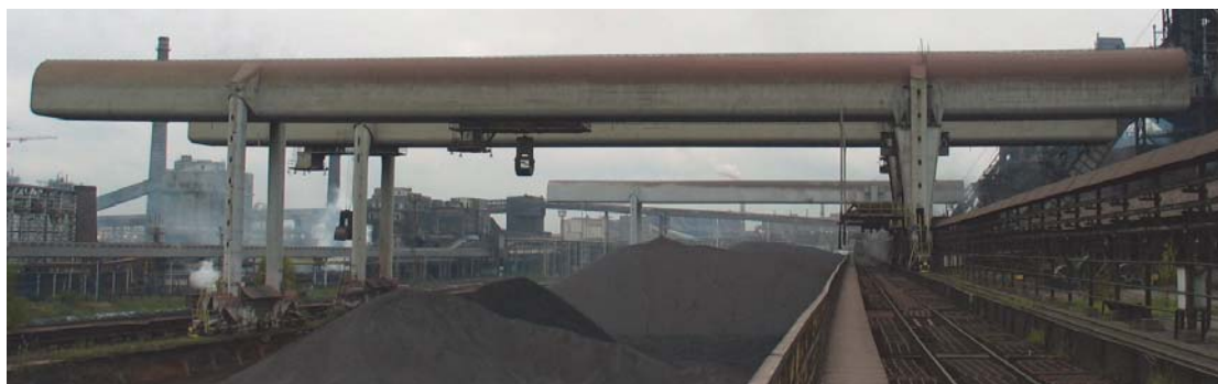
Fig. 1. Gantry cranes of a coating structure
