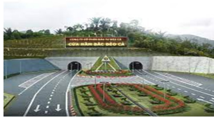
Fig. 2. Deo Ca traffic tunnel
