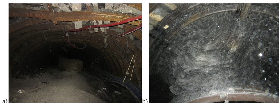
Fig. 10. The wedge of rock extrusion in the conditions of the “Belozerskaya” mine. Incline #1 (a) and Northern roadway (b) of l8 seam.
