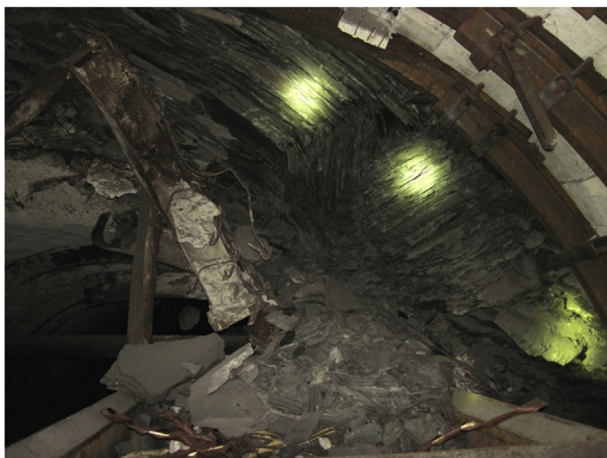
Fig. 12. The wedge of rock extrusion in the conditions of the “Sukhodolskaya-Vostochnaya” mine.
