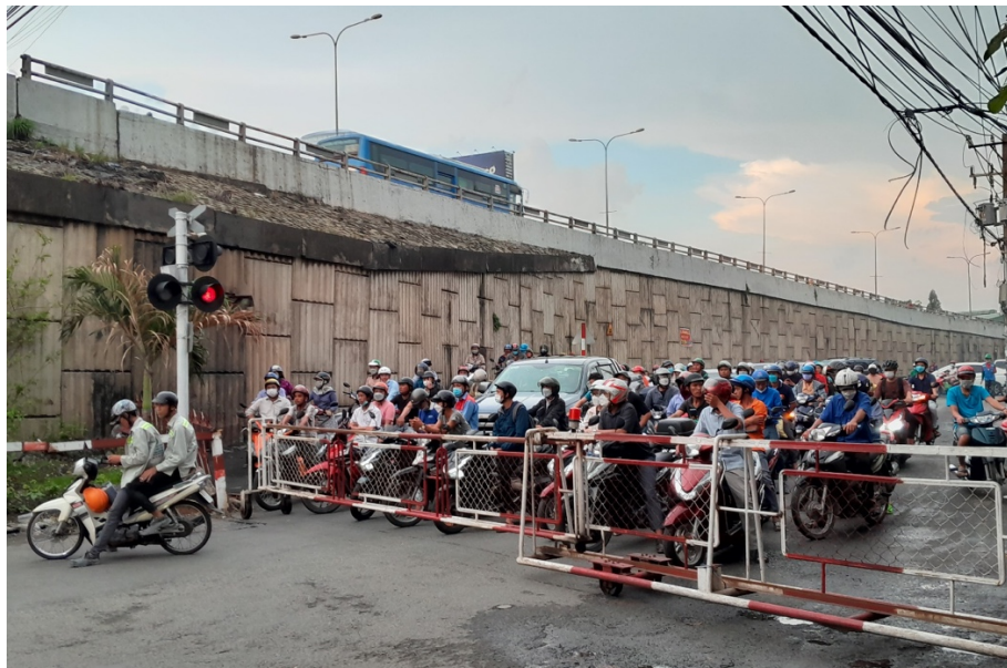
Fig. 3. A typical example of a solution used in the Saigon agglomeration: separated heavy vehicle traffic (on a viaduct and flyovers) and local traffic by roads crossing the railway infrastructure. Here: expectancy for the opening of the railway crossing in the northern part of Ho Chi Minh City, May 24, 2023
