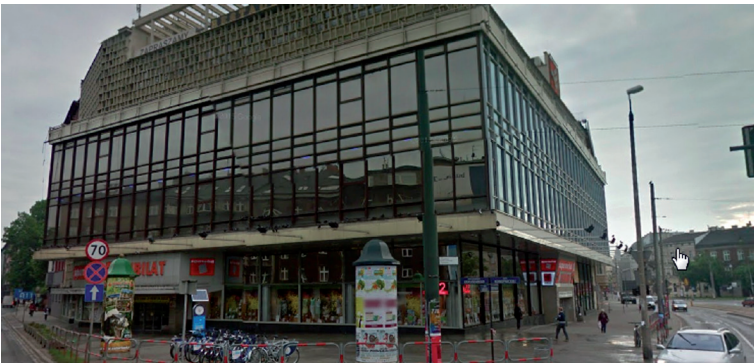
Fig. 8. Building at the intersection of Zwierzyniecka street and the Aleja Zygmunta Krasińskiego in Kraków
