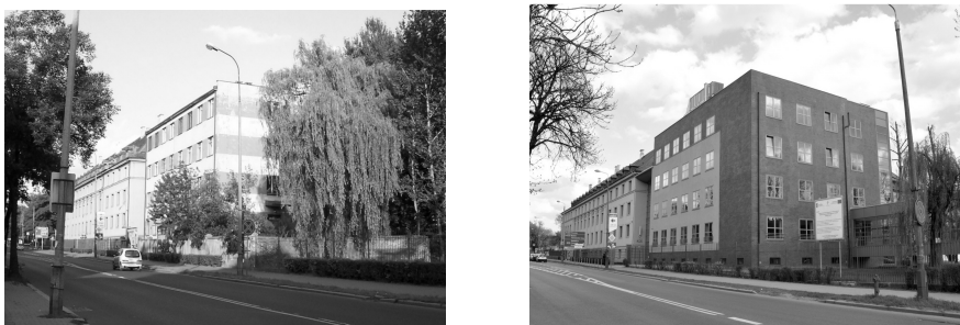
Fig. 13-14. The attitude of creative continuation – the reconstruction and extension of the Department of Organization and Management at Roosevelta Street 32 in Zabrze (former Military Command Replenishment). The design of the building sygn.1973 WBP, reconstruction 2006-2011, the authors of the project J.Witeczek, G.Nawrot, T.Wagner. The state before (2005) and reconstructed (2011) II . Photo by T. Wagner.
