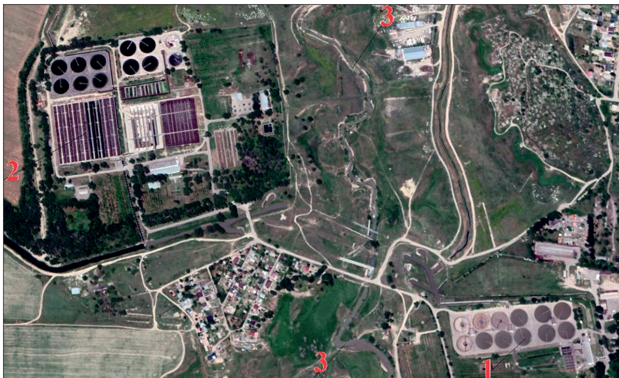
Fig. 1. Appearance of the sewage treatment plant: 1 – Mechanical treatment plant; 2 – Biological treatment plant; 3 – Bolshaya Almatinka River
