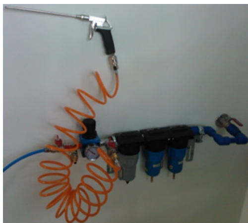
Figure 2. The filter system
